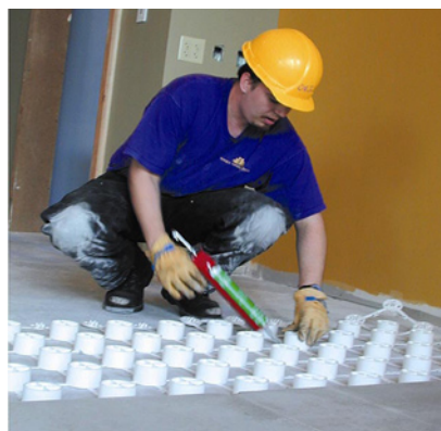
Applying Modular Base
