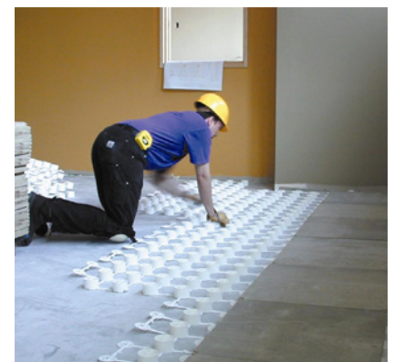
Installing Access Panels on Base
